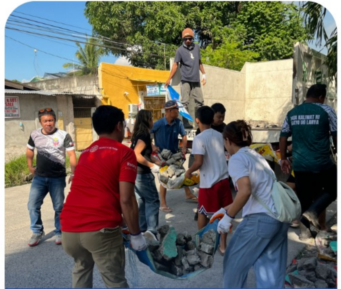
RESTORING HOPE. RACMD and GENSAN Council for Rotaract Clubs clear debris to prepare the school premises for learners.
